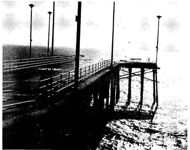
Figure 5. Abrupt end of Huntington Beach Pier photographed 20 January 1988. The seaward 250 feet of pier and "The End" Cafe were washed away Sunday evening 17 January 1988.
