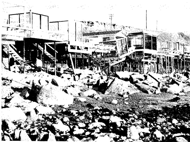
Figure 6. The trailer park at El Morro Beach suffered extensive damage to pipe pilings that support the trailer platforms. The entire cove area was stripped of sand.
