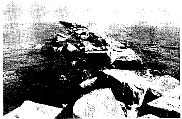
Figure 9. Damage of San Pedro breakwater.
