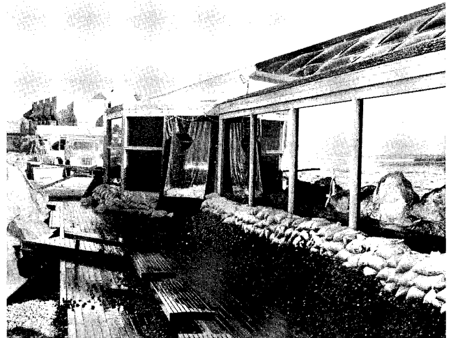
Figure 8. Wave overwash flooded the Chart House and other restaurants in Cardiff and along the shoreline in North San Diego County. Note cobbles thrown shoreward against the building.
