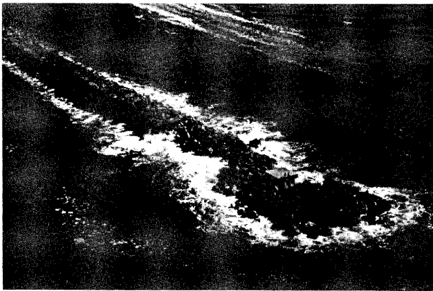
Figure 11. Damage to the head of the north jetty at Mission Bay, San Diego.
