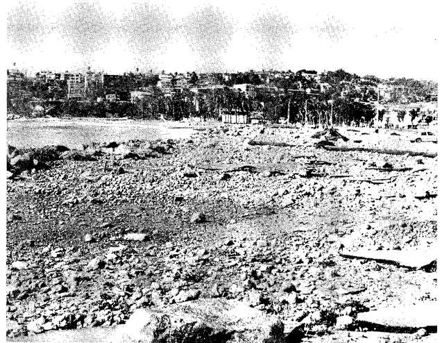
Figure 4. Photo showing overwashed and destroyed parking lot at Cabrillo Beach located at the western root of the San Pedro Breakwater.
